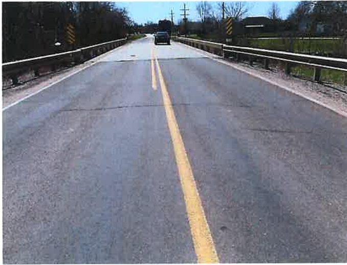
ROADWAY LOOKING SOUTH
