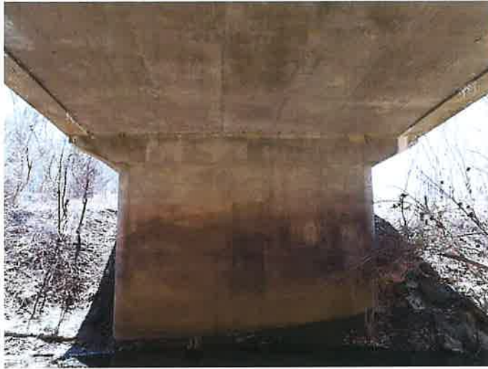
LOOKING SOUTH UNDER CENTER SPAN
